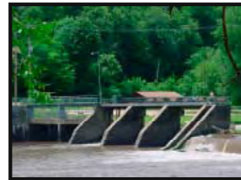
Oakland Mills Dam
